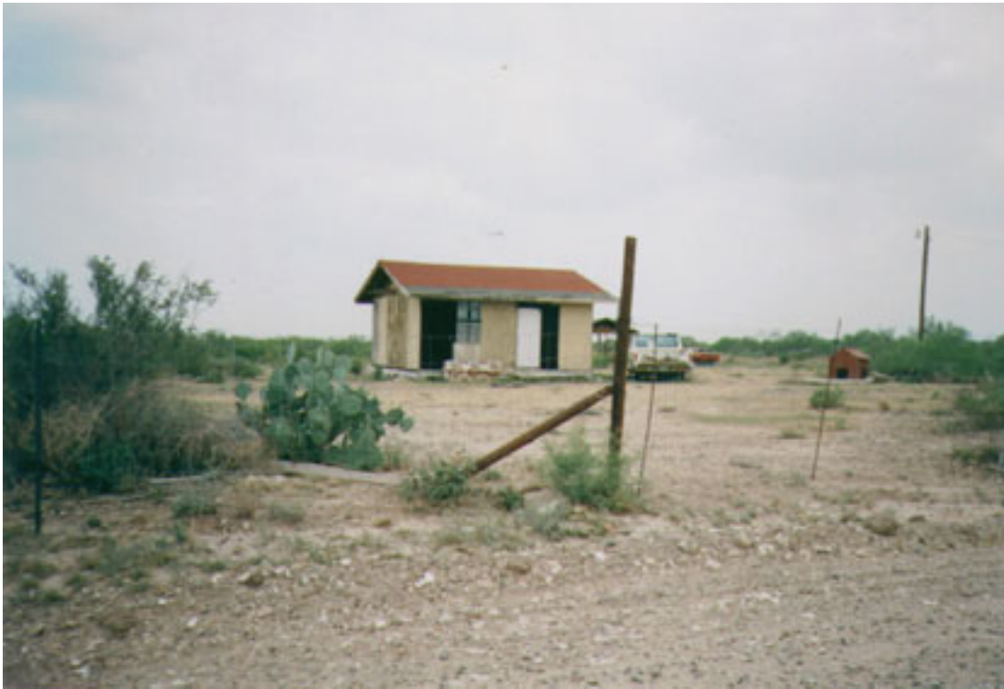
Figure 2. Home in Webb County, Tx Colonia Neighborhood
